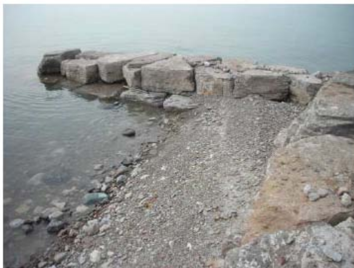
Figure 5.8 Small Armour Stone Groyne Installed on Lake Ontario
