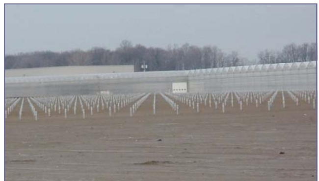
Setting posts for new greenhouses
