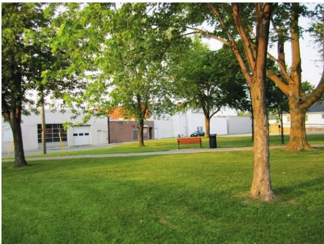
Figure 12. Rear facades facing public spaces should be upgraded.
