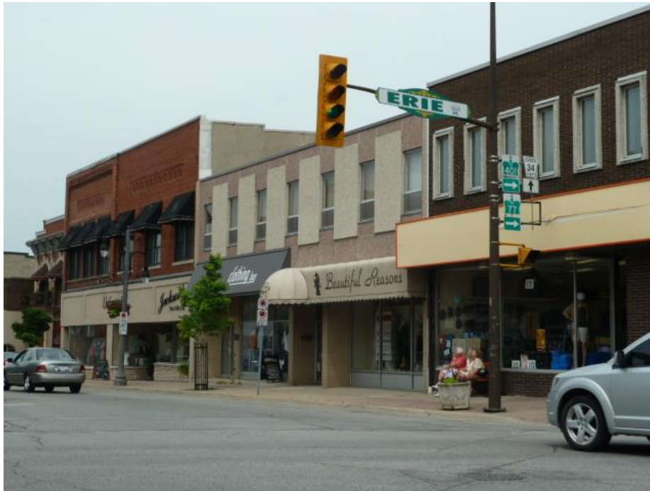
Figure 16. Two-storey to three-storey building heights ensure continuation of the 'street-wall'.
