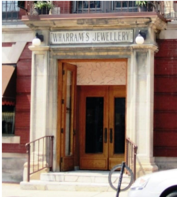
Figure 10. Feature entrance with doors, glazing, steps, should be preserved.
