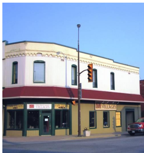
Figure 21. Permanent awnings built into the design of the building.
