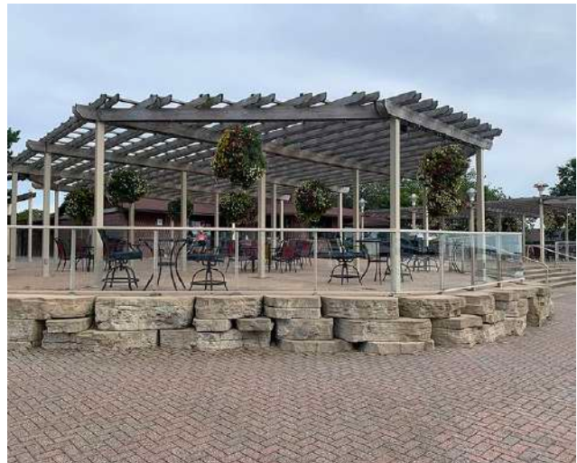
figure 63. Lakeside Marina patio and building
