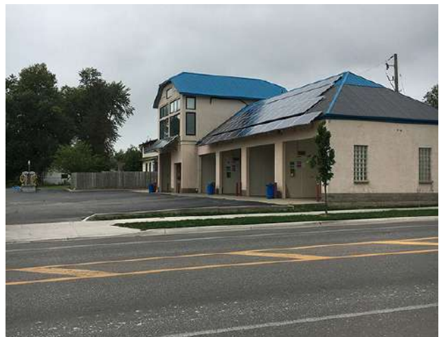
figure 71. 377 Erie St., looking northwest
