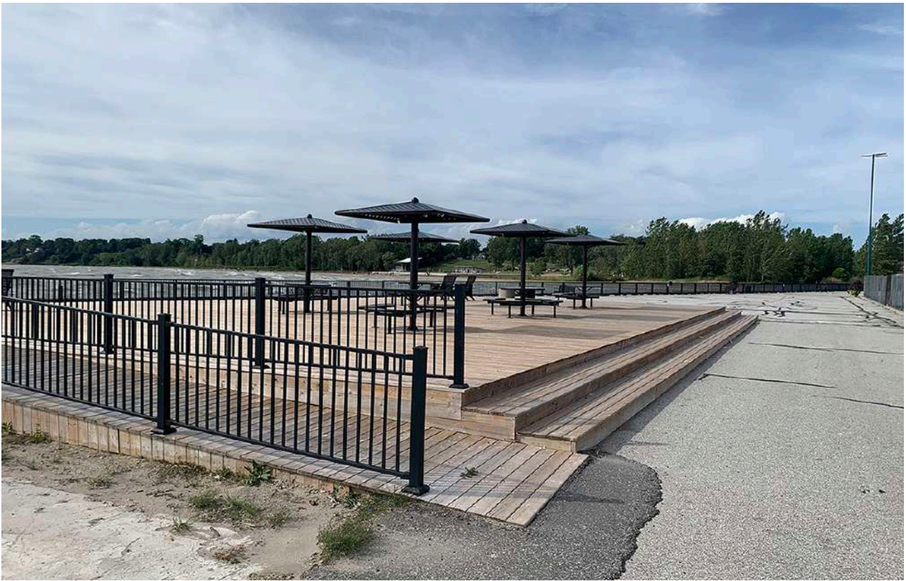
figure 32. Pedestrian Pier (Leamington Dock)
