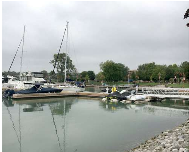
figure 62. Lakeside Marina docks, looking northwest
