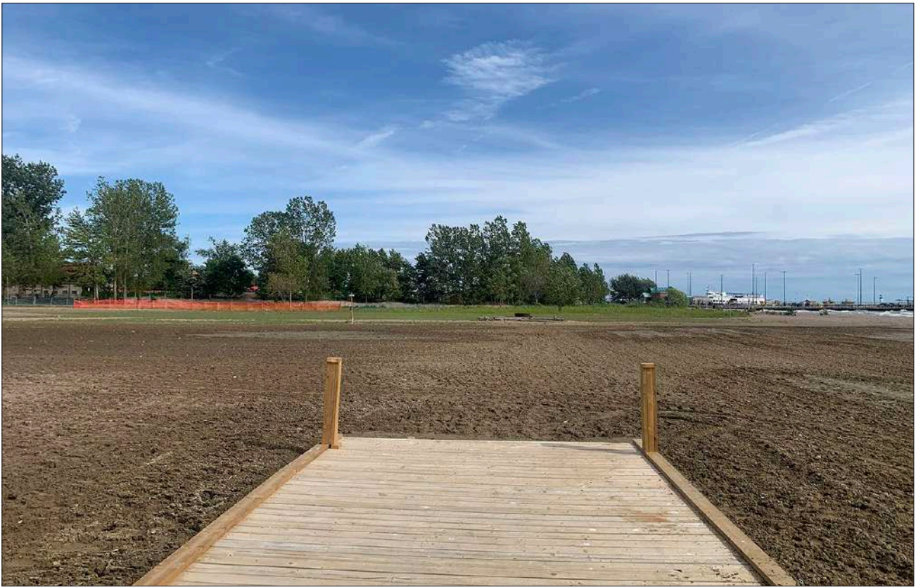
figure 90. The end of the boardwalk below Seacliff Park, looking east
