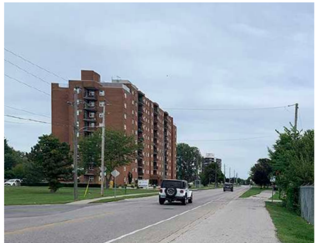
figure 70. Robson Road, looking east towards Lakeview Towers
