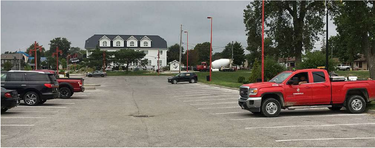
figure 31. Municipal Parking Lot, looking north
