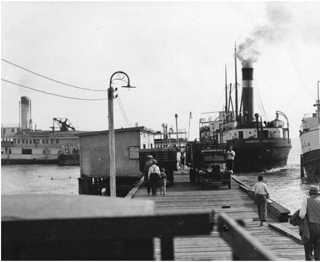
figure 34. Opening day at Leamington dock, September 1933
