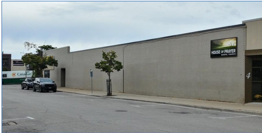
Picture 40: West side of Queens Avenue at Talbot Street
