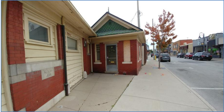
Picture 16: The 'Gregory Building', North Side of Mill Street
