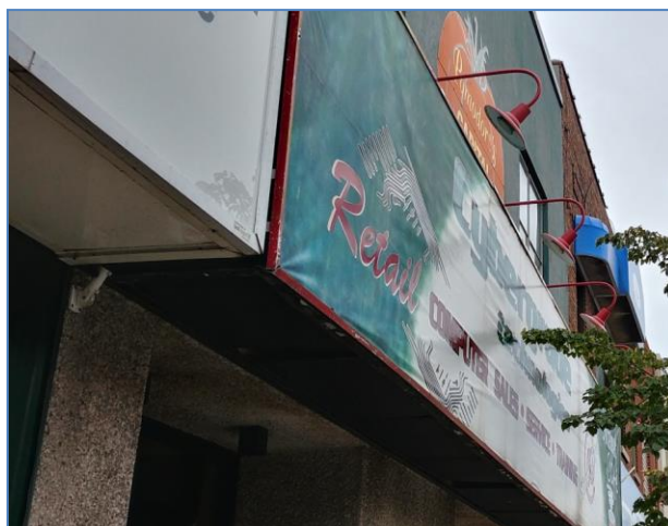
Picture 39: Existing Storefront Signage
