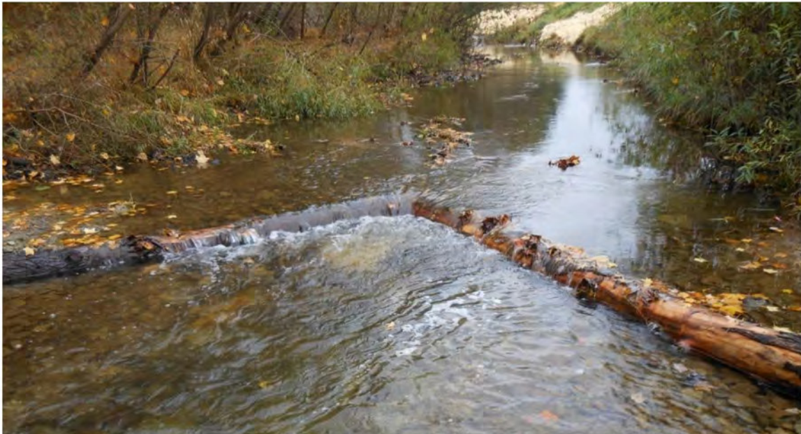
Figure 10 - Example of Timber Cross Vanes
