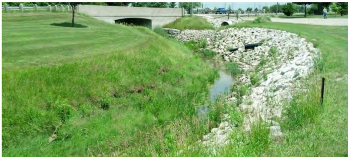
Figure 8 - Example of Drain Bank Restoration and Erosion Protection
