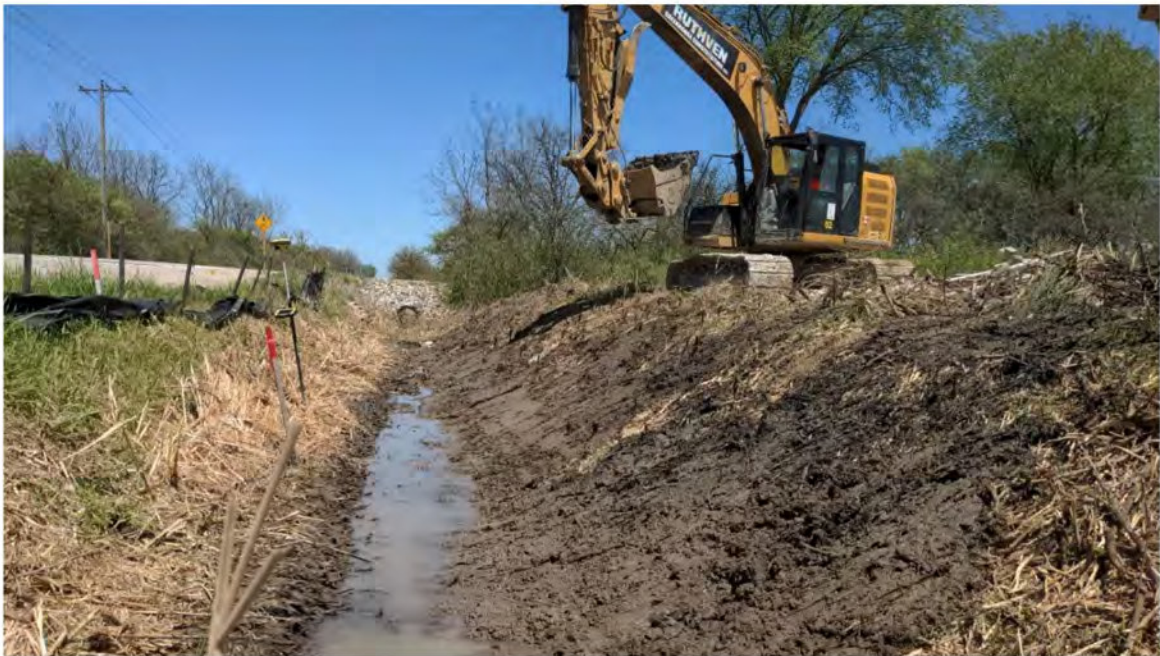
Figure 7 - Example of Drain Sediment Removal
