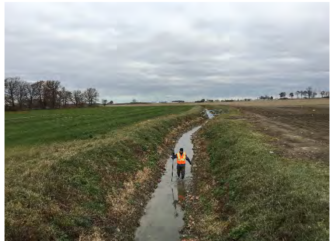
Photo 1: (SC – 7) Silver Creek Drain looking downstream from Mersea Road 7 culvert.
