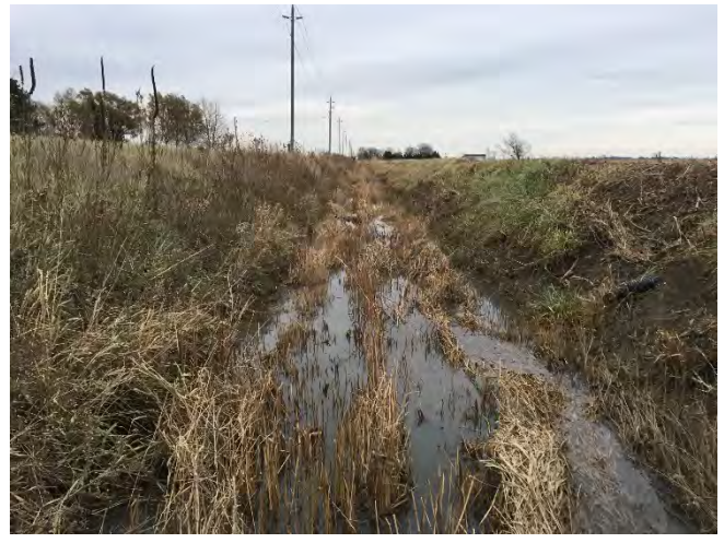
Photo 12: (BC – 14) Big Creek (9 th Concession road drain) parallel to Essex County Road 14 (on left side of photo), looking downstream. Approximately 1 km East of the intersection with Hwy 77.
