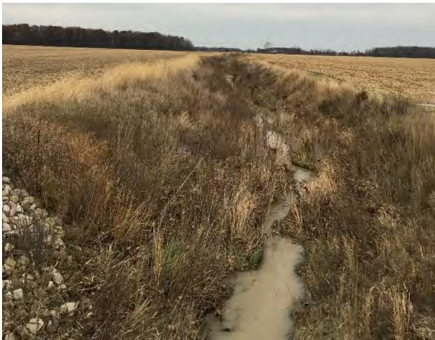
Photo 11: (BC – 10) Big Creek looking downstream from Mersea Road 10 culvert, notice the low flow sinuous channel that has developed.
