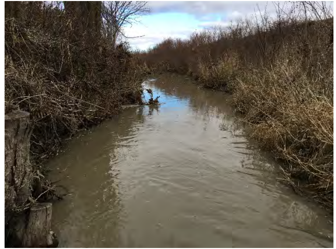
Photo 2: (SC – 8) Silver Creek Drain looking downstream, approximately 200 m North of Essex County Road 8.
