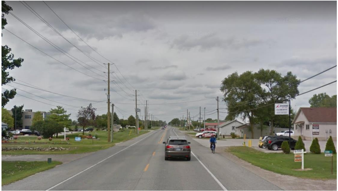
Looking north on Highway 77 showing cyclist travelling southbound on paved shoulder.
